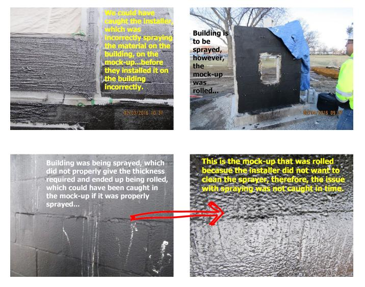
We have several projects where we rolled on the AVB on the mock-up because the installer did not want to bring out the sprayer and we have had issues with the installation that could have been caught on the mock-up early.
